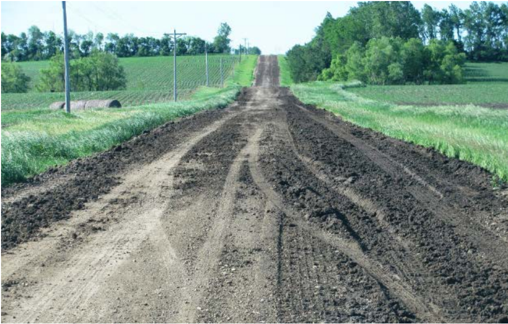
A road section heavily damaged during a wind energy construction project in wet conditions.
