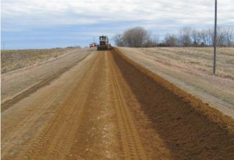
This operator had done an excellent job of completely windrowing and equalizing the new gravel . . . .
