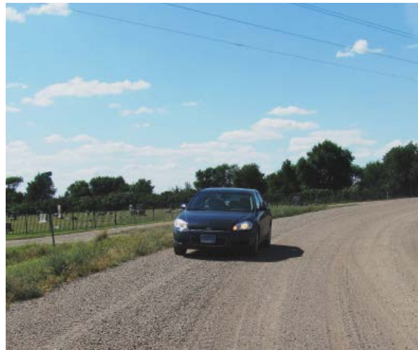
Well-shaped superelevation on a curve.
