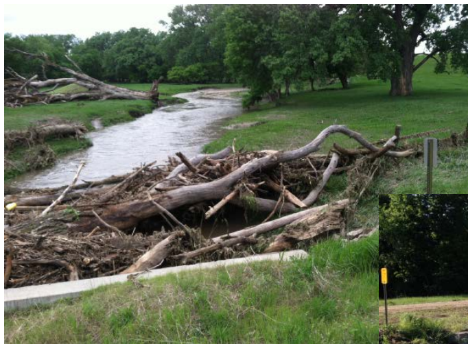
A large double box structure, completely plugged with debris after flooding and the same structure after debris removal and channel clean-up by a county maintenance crew.
